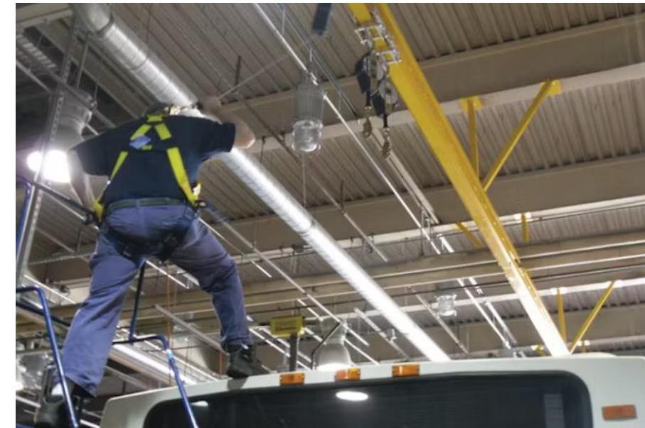
Source: Mass Transit, https://www.masstransitmag.com/rail/product/11151229/fall-protection-systems-rigid-rail-trolley-system
